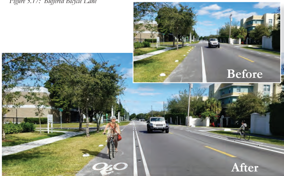
Figure 5.17: Buffered Bicycle Lane
