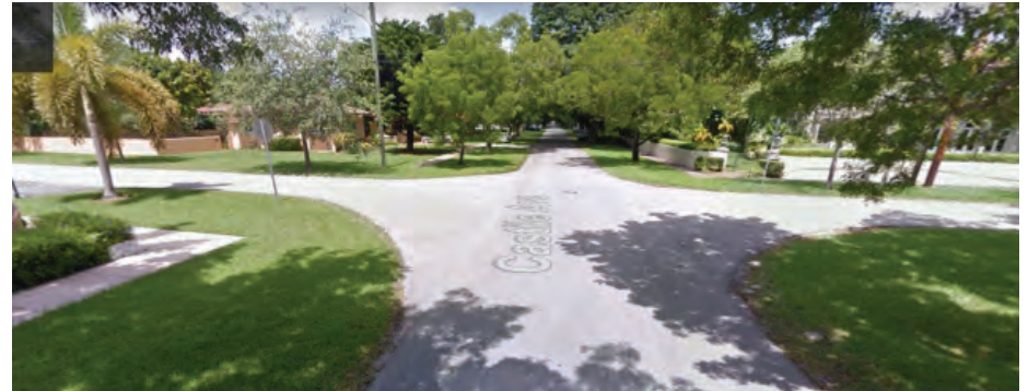
Intersection with missing and unconnected sidewalks
