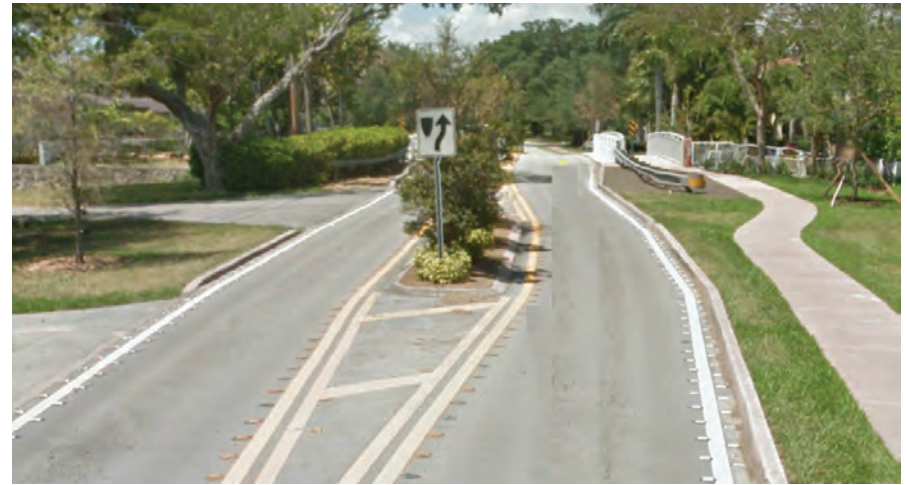
Figure 8.5: Existing Median Divider
