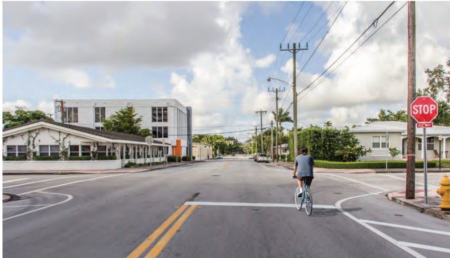
Figure 5.37: Salzedo St. Existing Conditions
