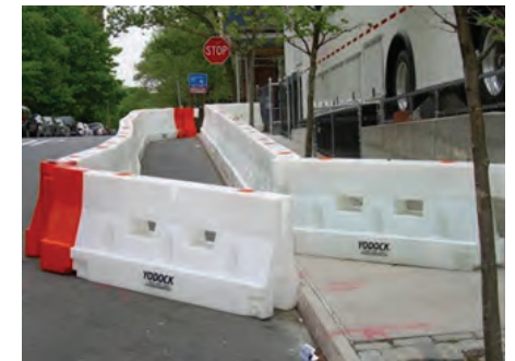
Suitable accommodation of pedestrians in a work zone.
