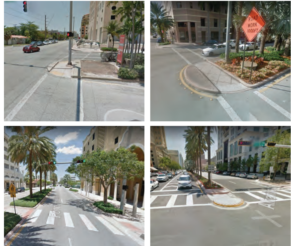
Figure 4.22: Existing Pedestrian Refuges in Coral Gables
